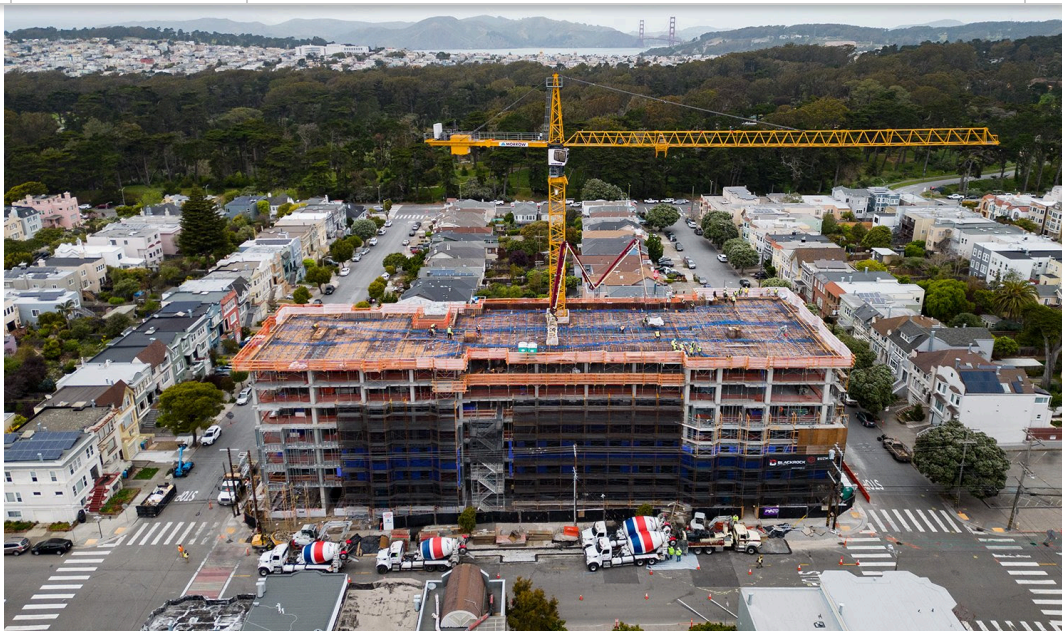
Photo of 2550 Irving taken during it's construction.
