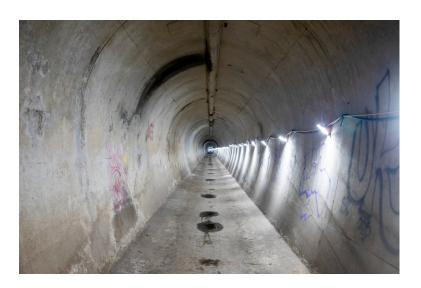
The picture above is of the Lake Merced Tunnel which is 14'0" diameter and travels 1.6 miles. See red line in Sewage Piping Diagram
