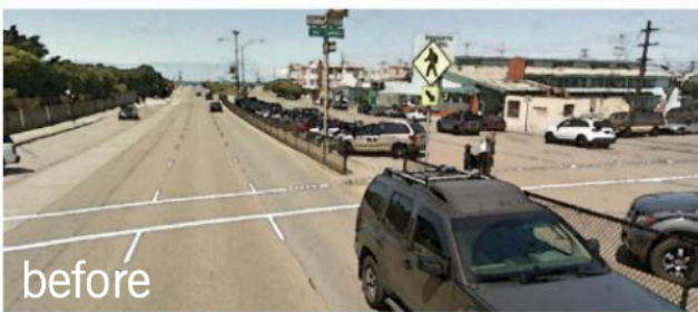
Figure V-4a: Existing Sloat Blvd = Parallel and Diagonal Parking + 3 Driving Lanes + Diagonal Parking + 3 Driving Lanes
